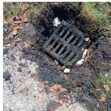
Pic of drain
