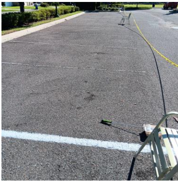
Pic before repainting
