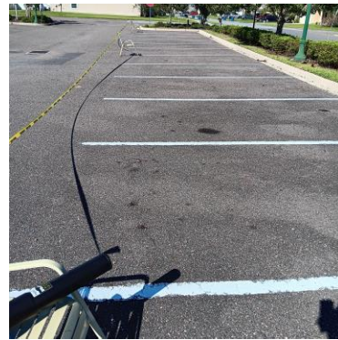
Pic after the repainting
